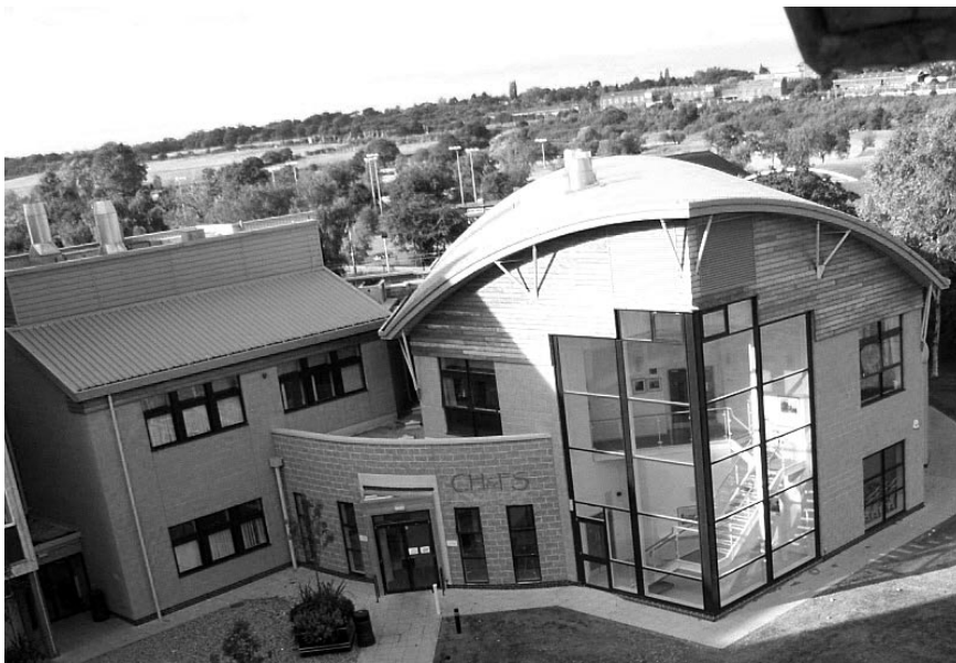
(Left) The CH&FS new building, designed for the delivery of industry-standard training and education.
